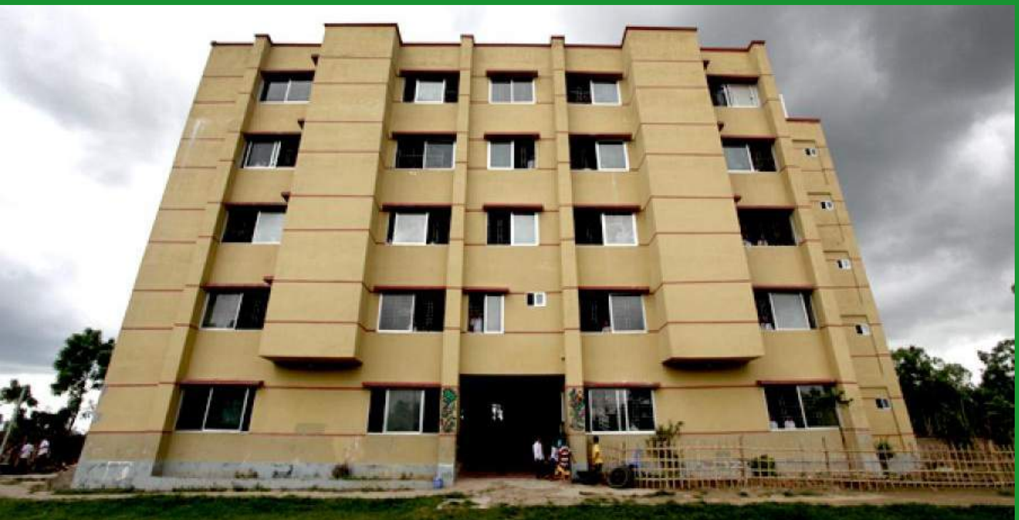
AMCC main building in Panchagarh
